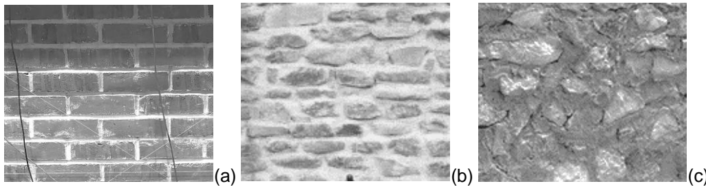
Figure 1. Typical masonry patterns: (a) regular clay brick masonry, (b) cut stone with good bond, (c) irregular stone masonry, with pebbles, erratic and irregular stone units.
