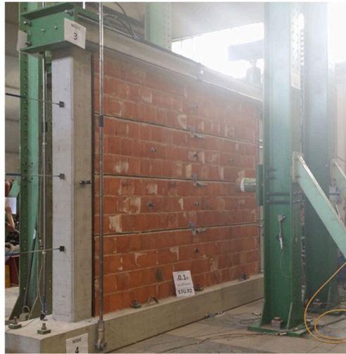
Figure 2. Masonry wall with horizontal and vertical rubber joints tested within INSYSME project.
