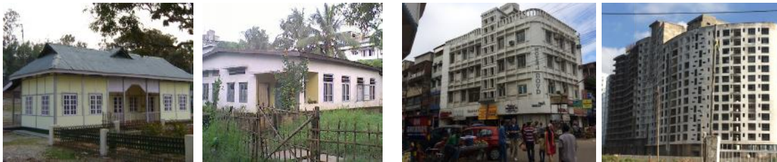
Figure 5. Example of existing and predominant building typology classes in Guwahati city: (a) Traditional Assam-type (Ikra) house; (b) Confined masonry building; (c) Older (non-ductile) RC frame building; (d) Ductile RC frame building under construction
