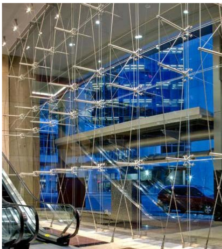
Figure 3–Example of bow truss tension cable glazing system
