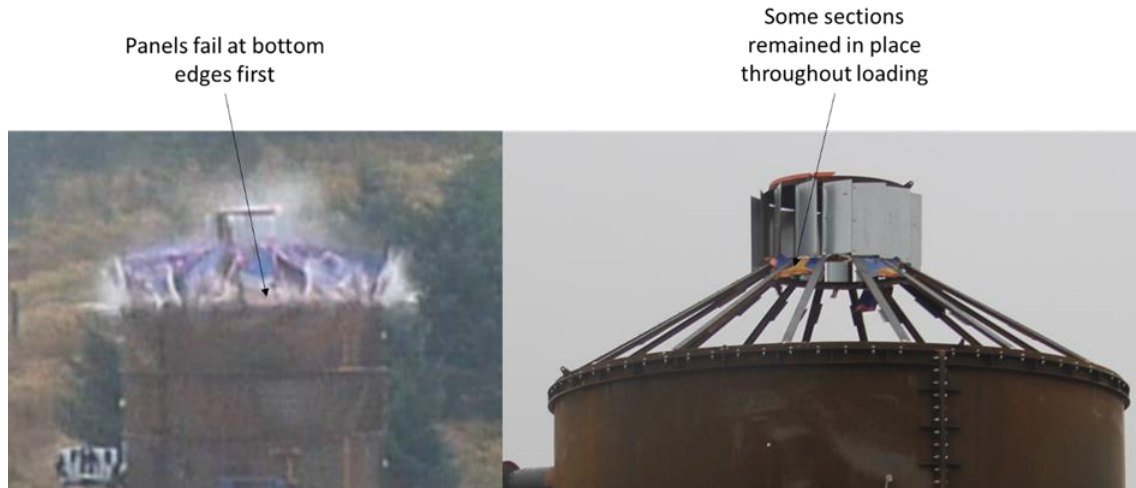
Figure 13 – Frangible panels during and after explosion event
