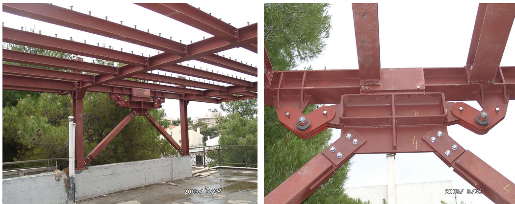
Figure 4. Residential building. General view of damper bracing and dampers detail.
