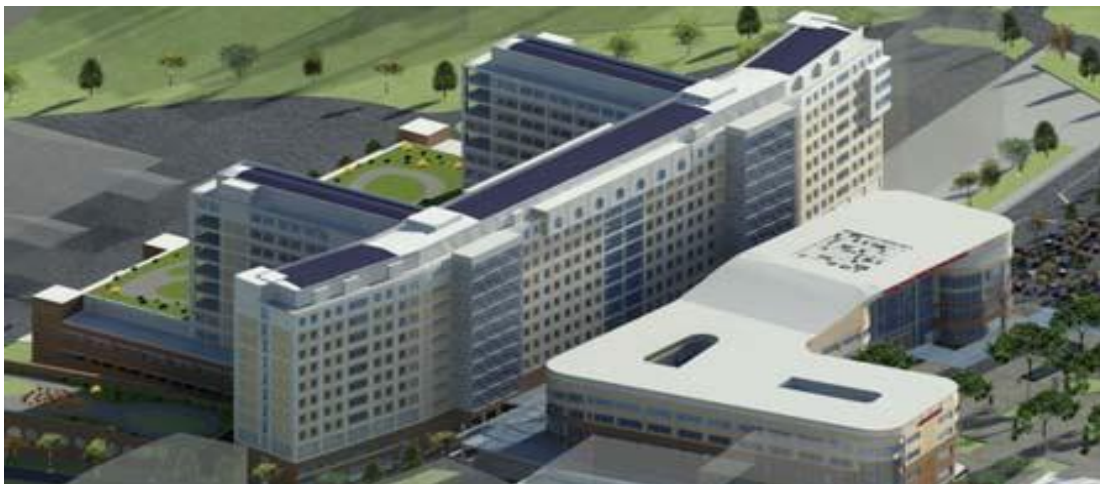
Lutfi Kirdar Hospital, 3 Million Sq. Ft, Turkey
