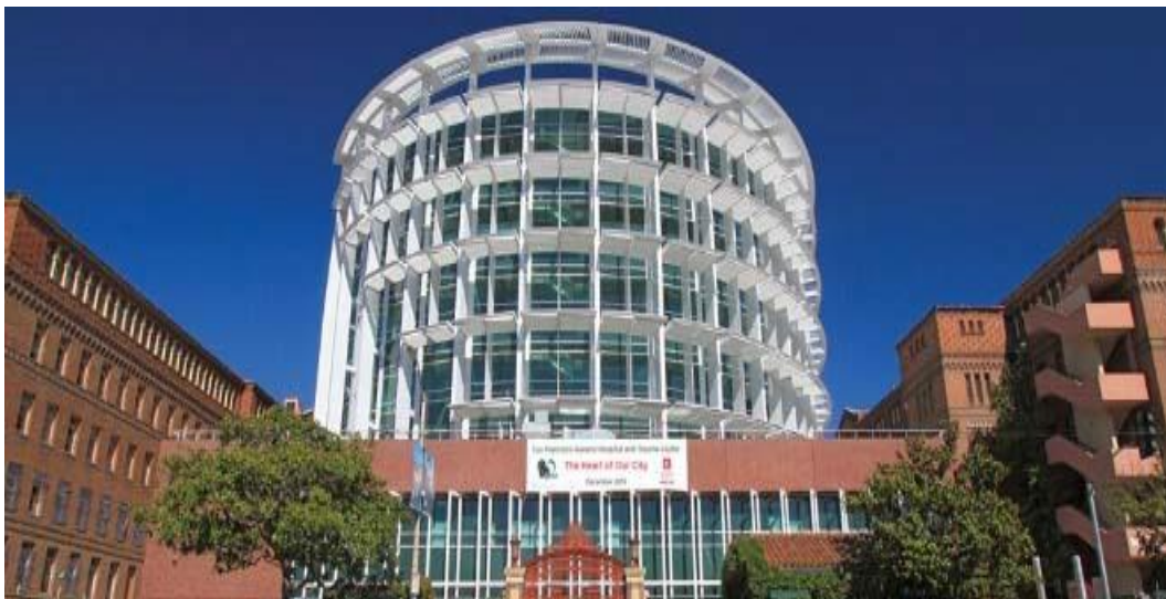
San Francisco General Hospital, San Francisco, California
