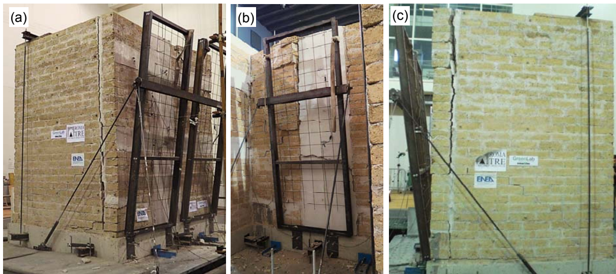
Figure 5. Damage pattern induced by shake table tests on the specimen strengthened with SRG: vertical cracks at the corner separating the façade from the side walls (a), damage in the internal side of the front wall (b), and damage in the side walls (c).
