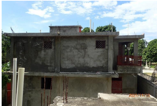
Figure 3. Example of unreinforced hollow block masonry with concrete slabs.
