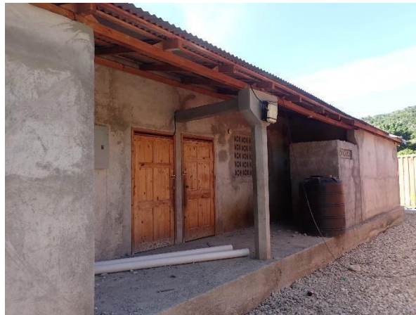
Figure 4. Example of unreinforced hollow block masonry with light roof.
