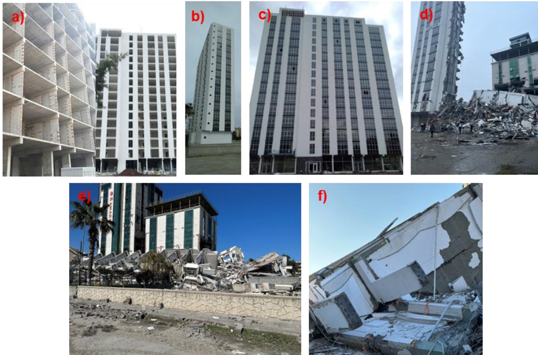
Figure 10. Example of post-2000 building collapses; a), b), and c) Before the earthquakes; d) After first earthquake; e) and f) After second earthquake.
