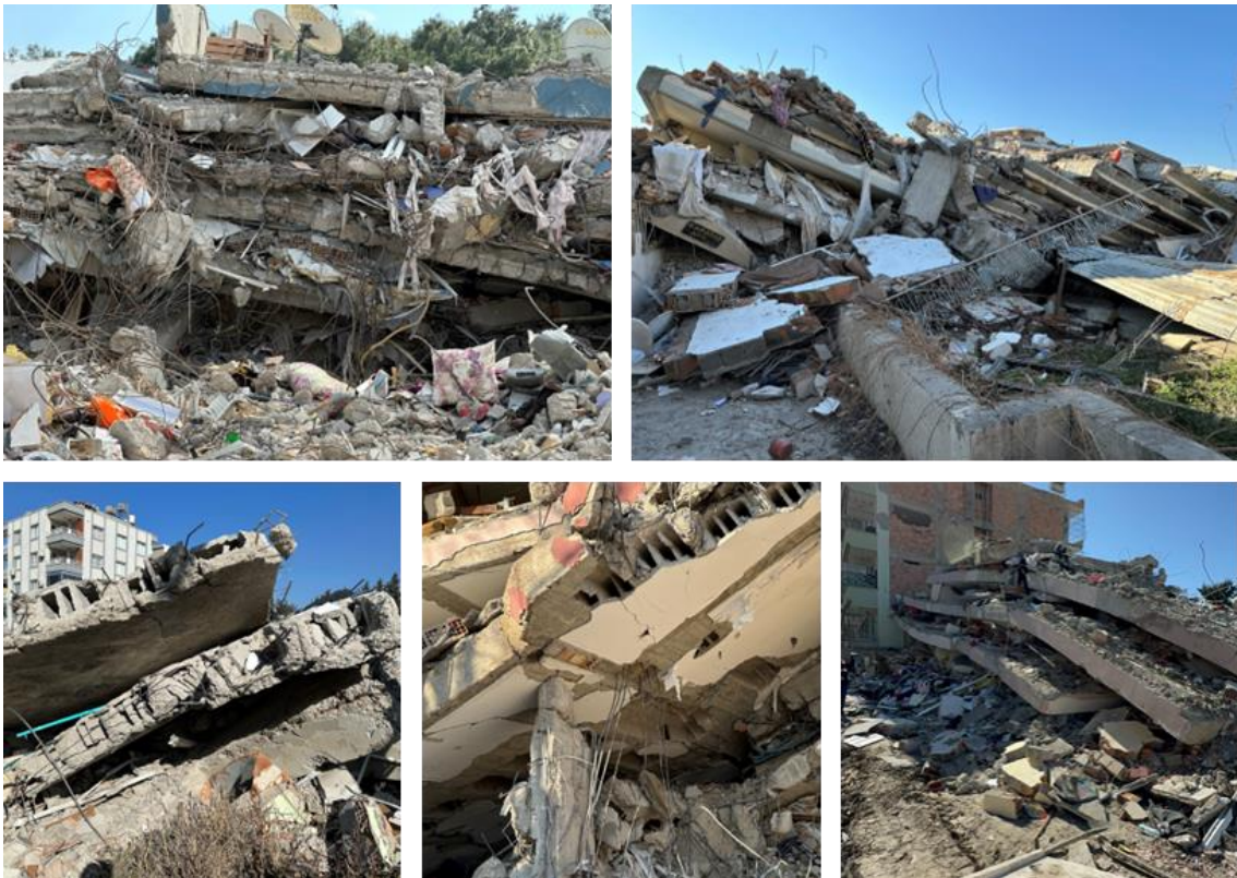
Figure 7. Failures of buildings with ribbed slab.
