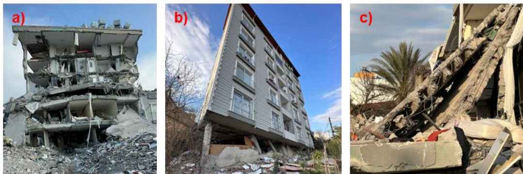
Figure 11. Illustration of collapses in post- 2000 buildings; a) Front view; b) Back view with softstorey mechanism; c) View of ribbed floor slab.
