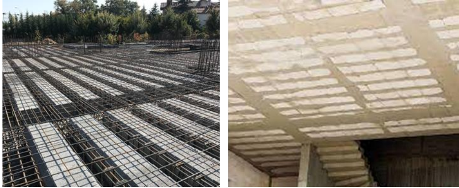
Figure 6. Examples of ribbed floor slabs construction.
