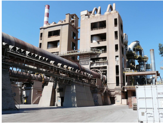
Figure 5. Preheater buildings for Lines 1 & 2 (Line 1 on the right).
