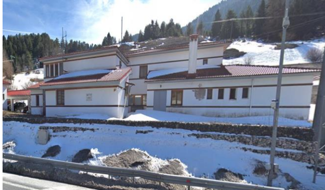
Figure 7. Operator control building.
