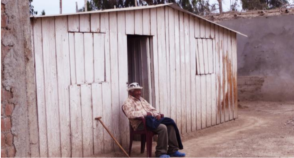
Figure 1. Non-modified transitional house in Peru after 5 years of use provided by TECHO. (Wagemann)
