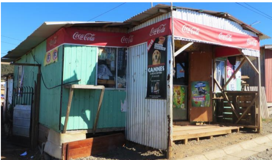
Figure 2. Example of a modified transitional house in Dichato, Chile, 2012. (Wagemann)
